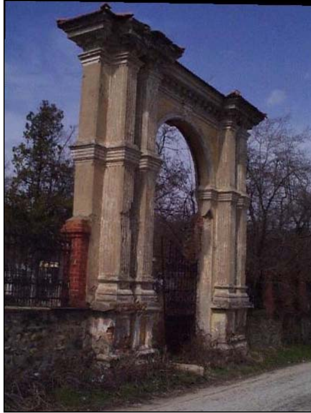
Photo 4.1: Arched entry of the Bukovo cemetery in Bitola
